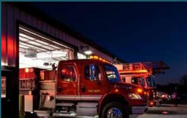
FIRE SERVICE STATION
