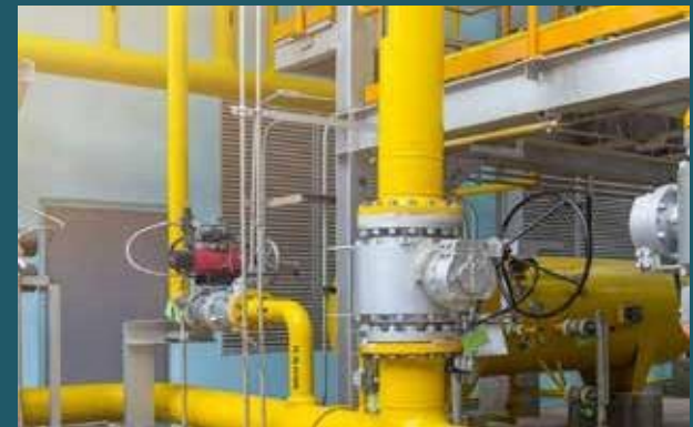
GAS TO HOUSE
